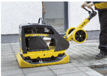
No breakage of paving stones
