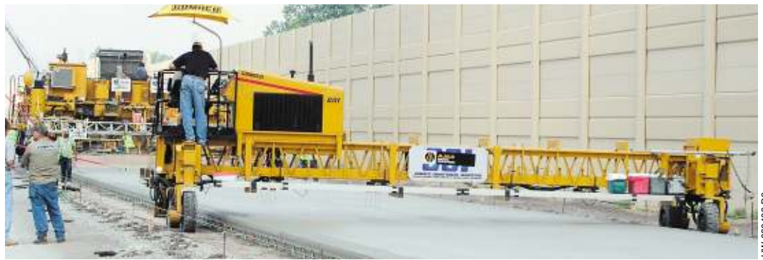
The GSI can operate off the same stringline as the paver. Here it is measuring smoothness directly behind the finishers.
