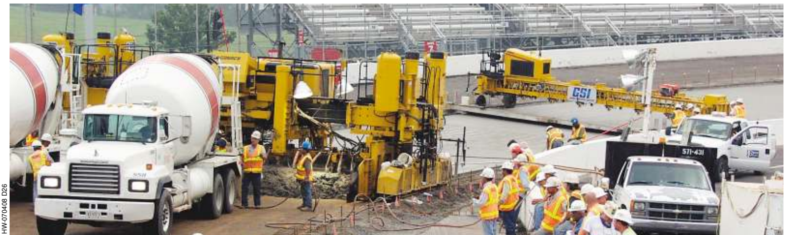
A new generation GHP-2800 paves the curve on the Martinsville Speedway in Virginia for NASCAR racing. A GSI follows the paver to check smoothness results.
