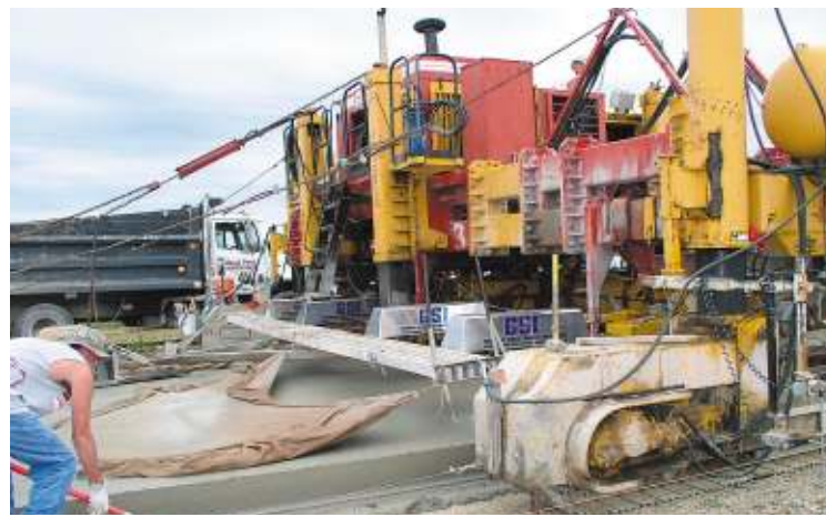
The GSI can operate off the same stringline as the paver. Here it is measuring smoothness directly behind the finishers.
