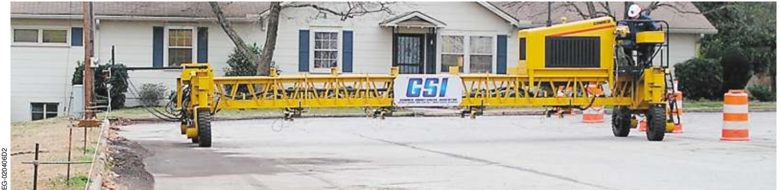
The GSI was successfully tested for repeatability by steering from stringline. The GSI was taken off line and returned to line for retracing. Similar traces revealed excellent repeatability by the GSI.
