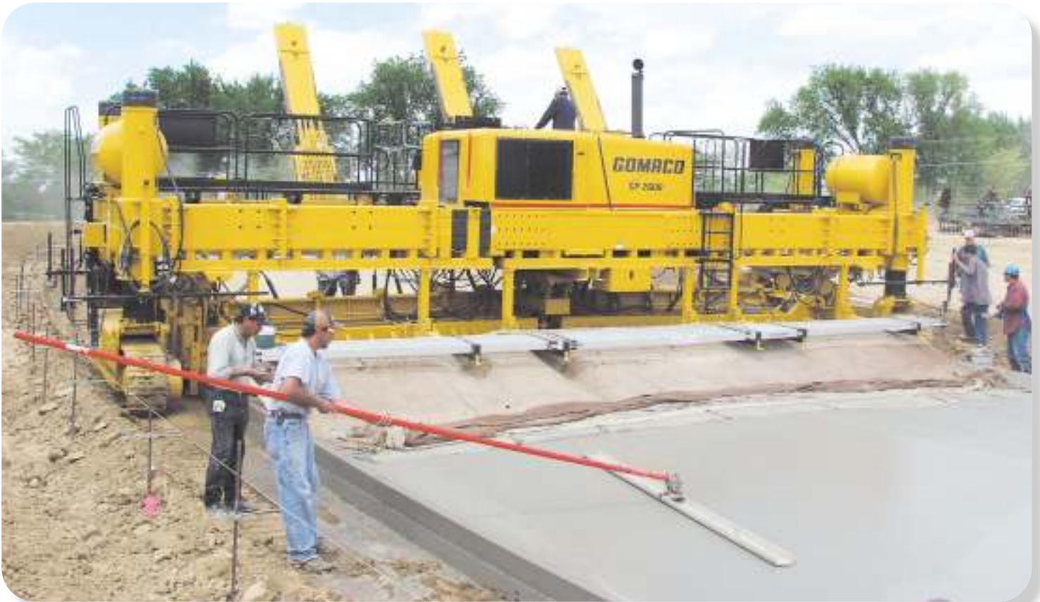
The two-track GP-2600 is slipforming a cul-de-sac with a 95 ft. (29 m) inside radius. This machine is equipped with three frame-mounted bar inserters. This street in Wayne, NE, is being slipformed full width with integral curb on both sides.
