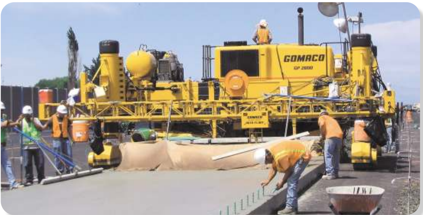
This versatile four-track GP-2600, equipped with the GOMACO Auto-Float® slipforms mainline paving in Salt Lake City, UT.
